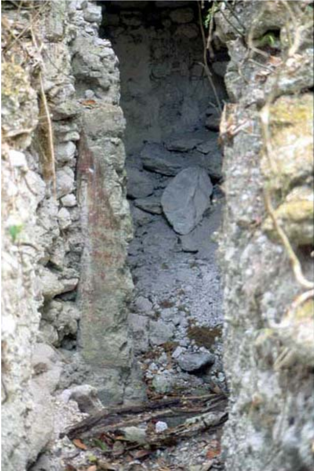
Figure 7. El Gallinero, looters' trench in Structure A-3, looking south.
