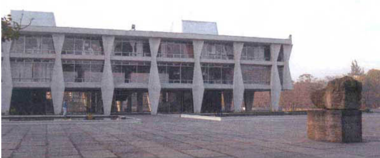
Figure 9. Another aspect of the monument's position in front of the USAC's Rectory Building.
