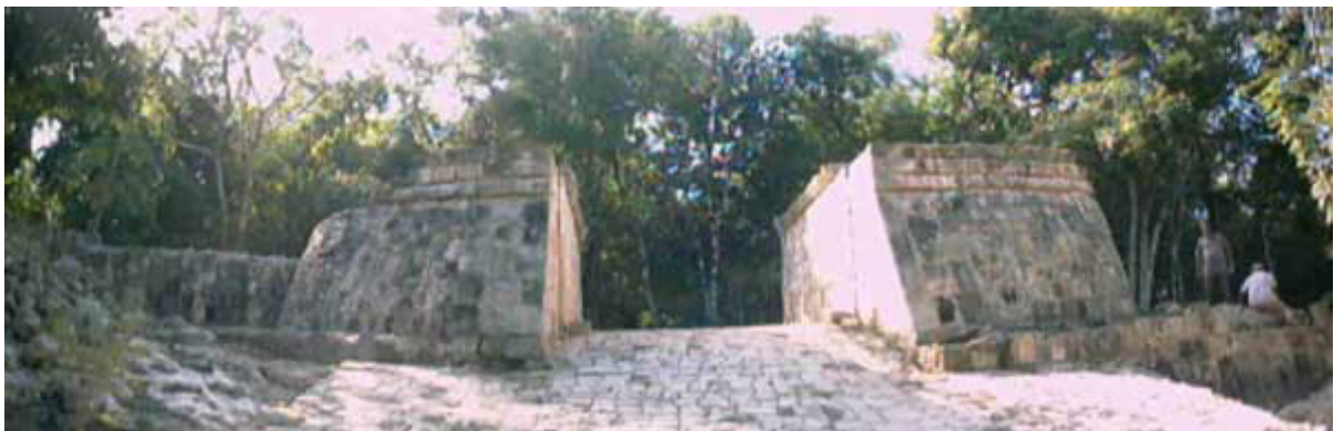
Figure 3. Structure 5C35, north façade.
