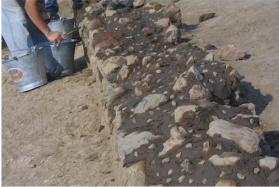
Photo 23. Consolidation of the walls.
