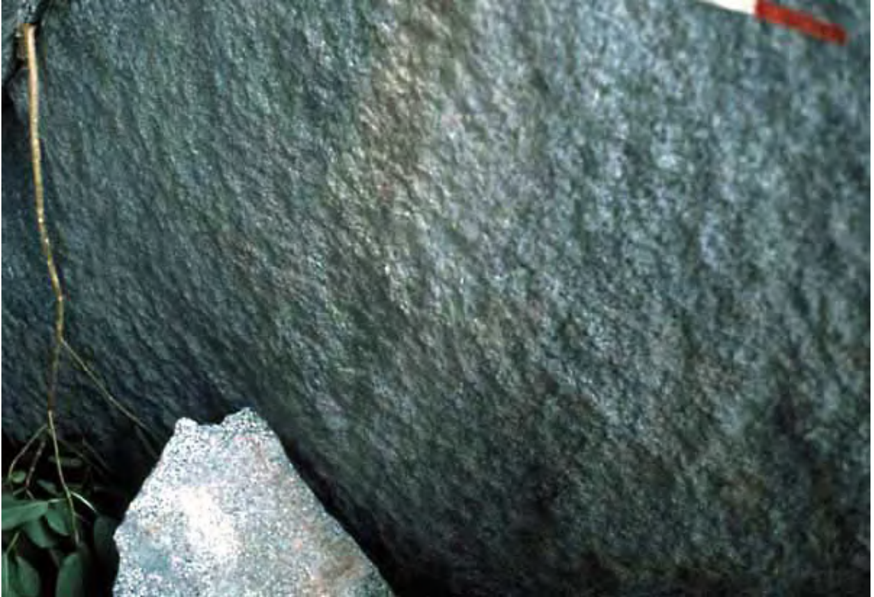
Slide 21: Sub-Area A-1, walls i-iv, details.
