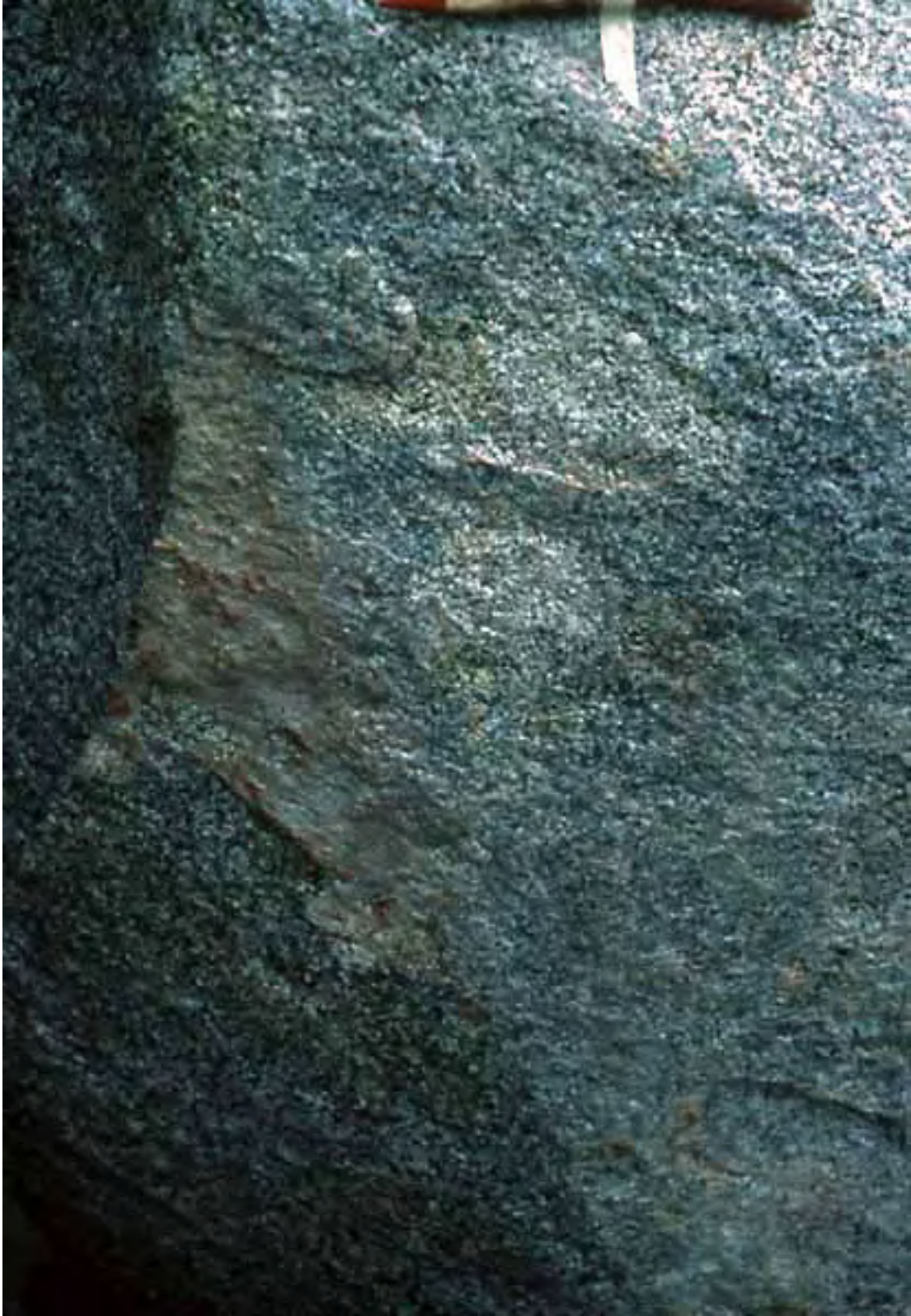
Slide 17: Sub-Area A-1, walls i-iv, details.
