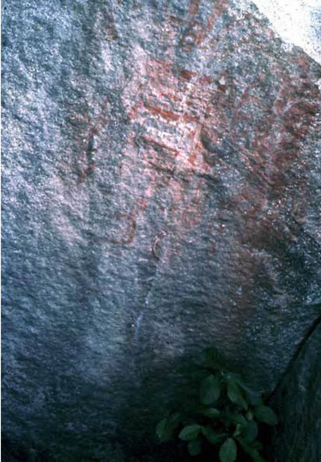
Slide 26: Sub-Area A-1, wall v, general and detail views.
