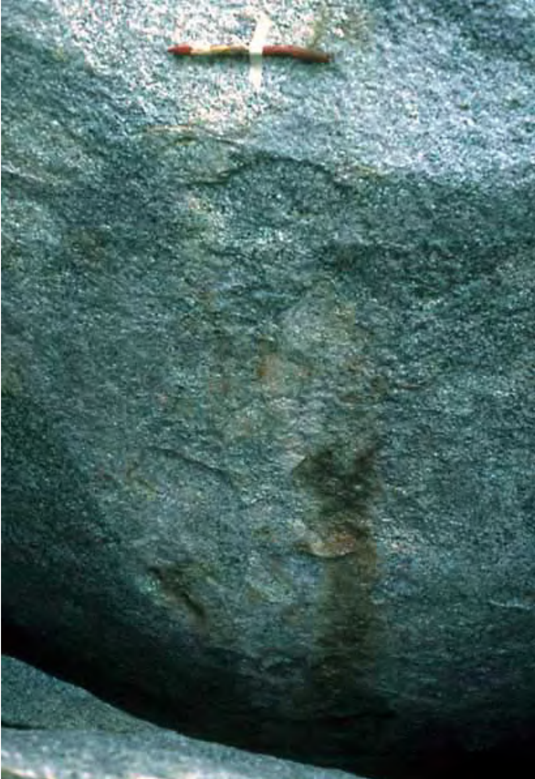
Slide 13: Sub-Area A-1, walls i-iv, details.
