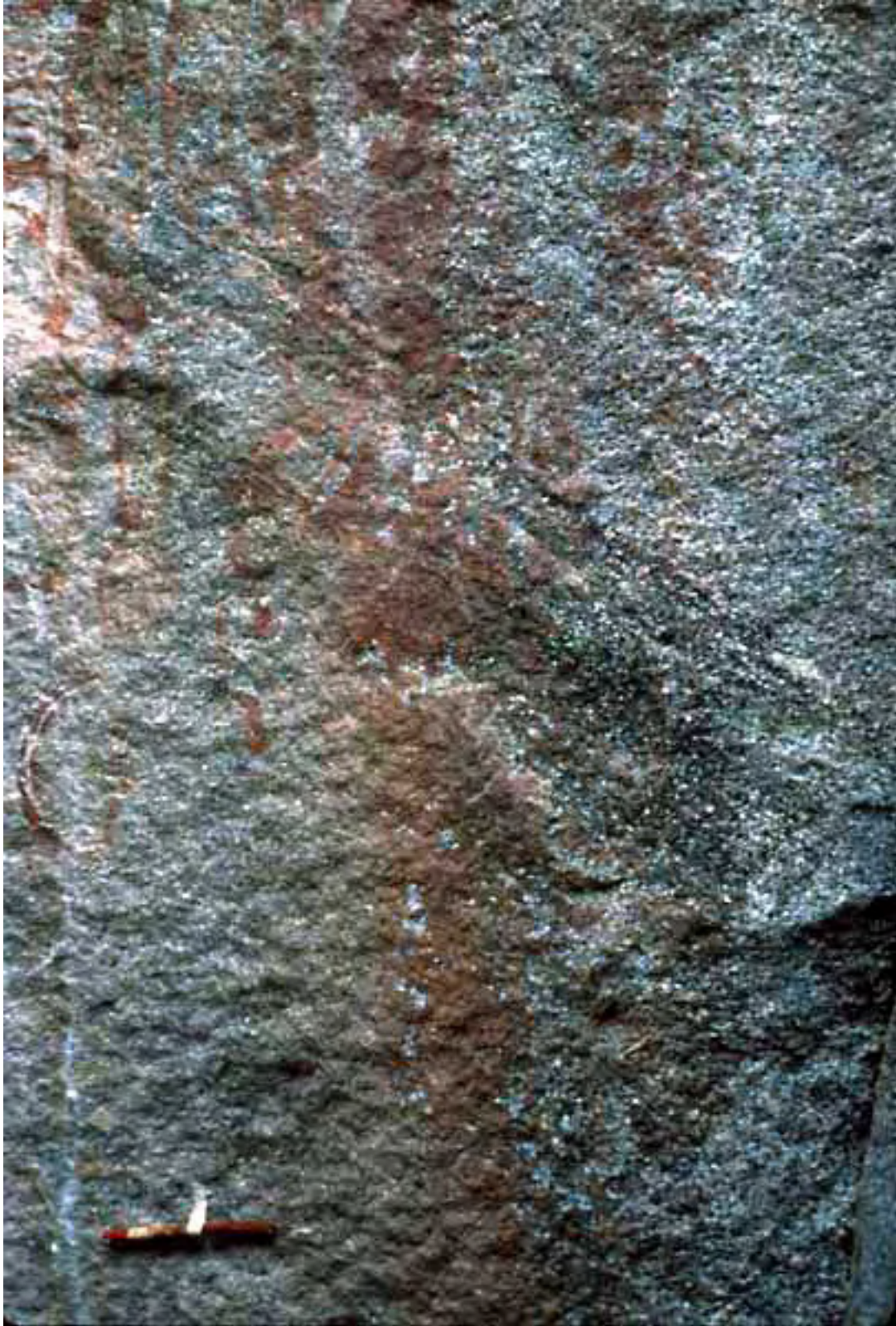
Slide 24: Sub-Area A-1, wall v, lower area.
