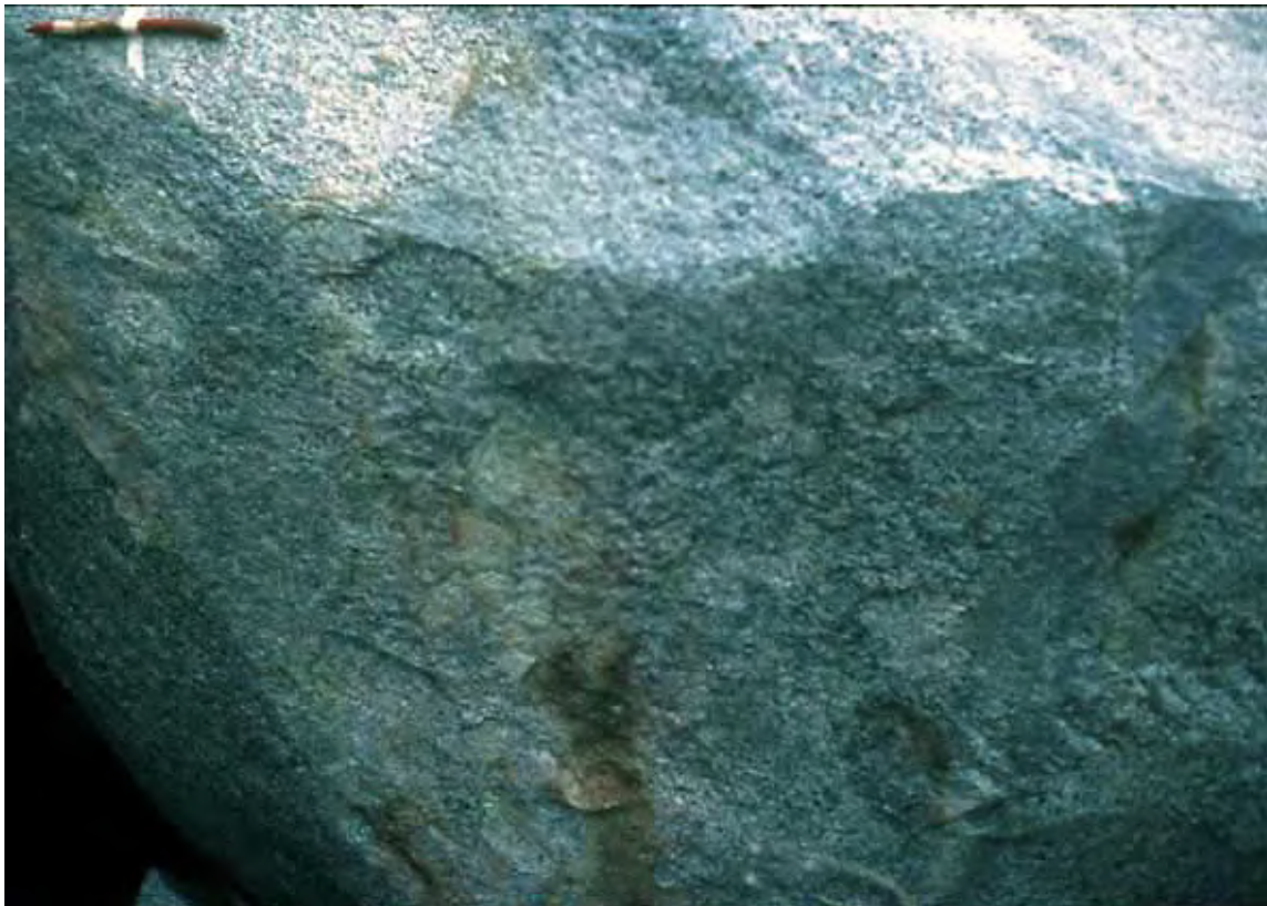
Slide 11: Sub-Area A-1, walls i-iv, details.
