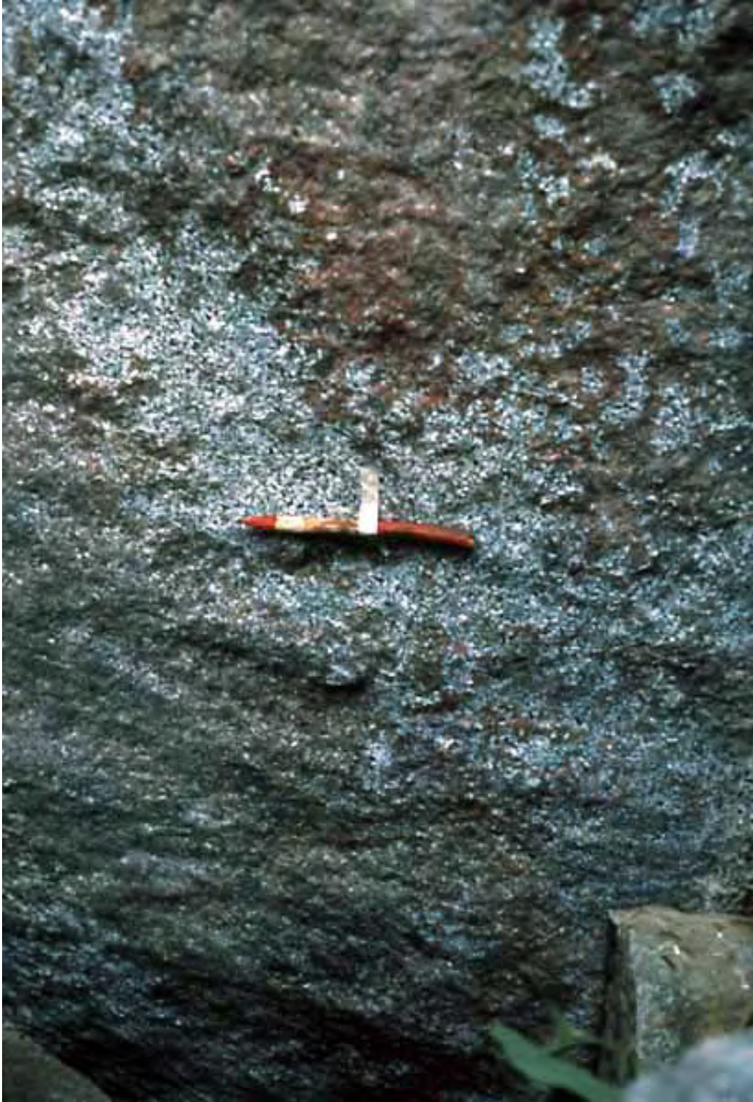
Slide 22: Sub-Area A-1, wall v, lower area.
