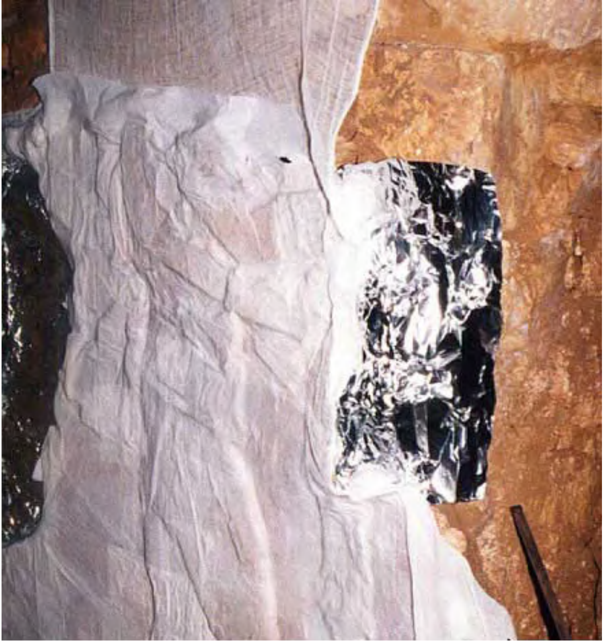
Photo 12. Preparing the stucco relief for detachment
