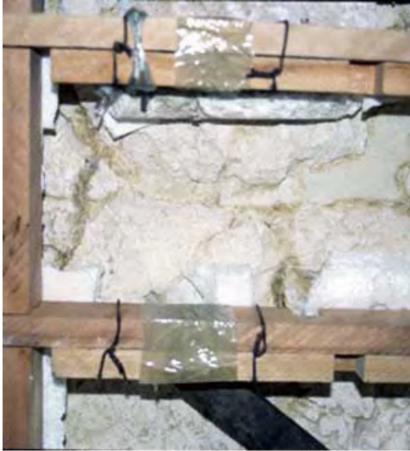
Photo 58. Repairs with ribs paste in the back
