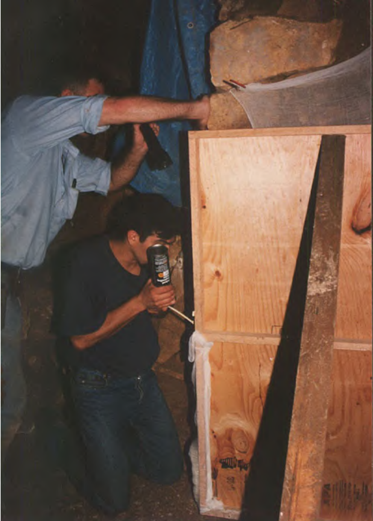
Photo 13. Injection of polyurethane foam
