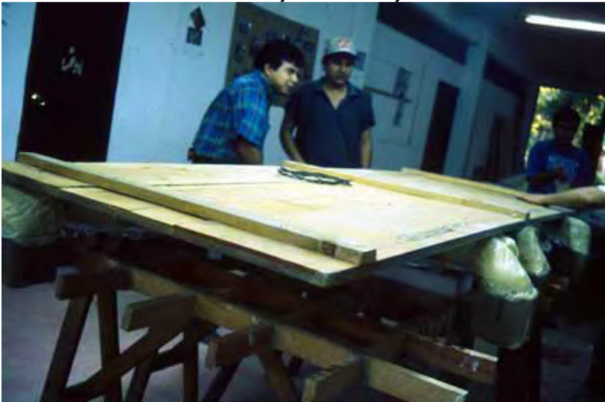
Photo 67. Placement of plank for turning over the stucco panel
