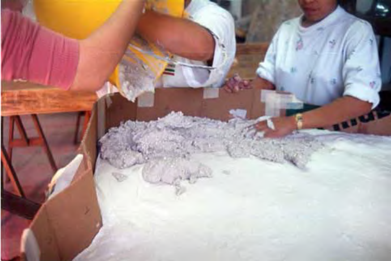
Photo 32. Application of plaster with polystyrene pearls
