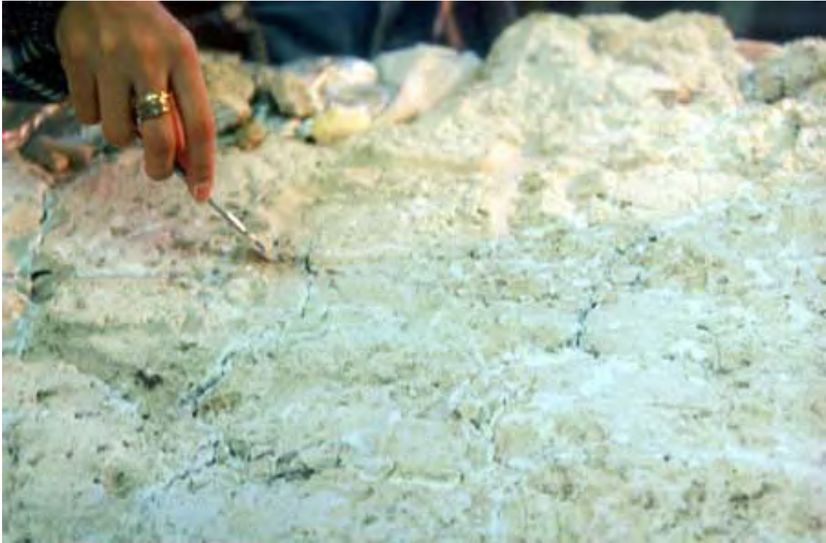
Photo 23. Consolidation of cracks and fissures on the reverse of the detachment
