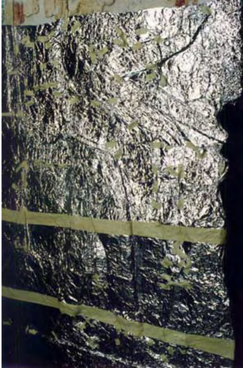
Photo 64. Protection covers with aluminum foil
