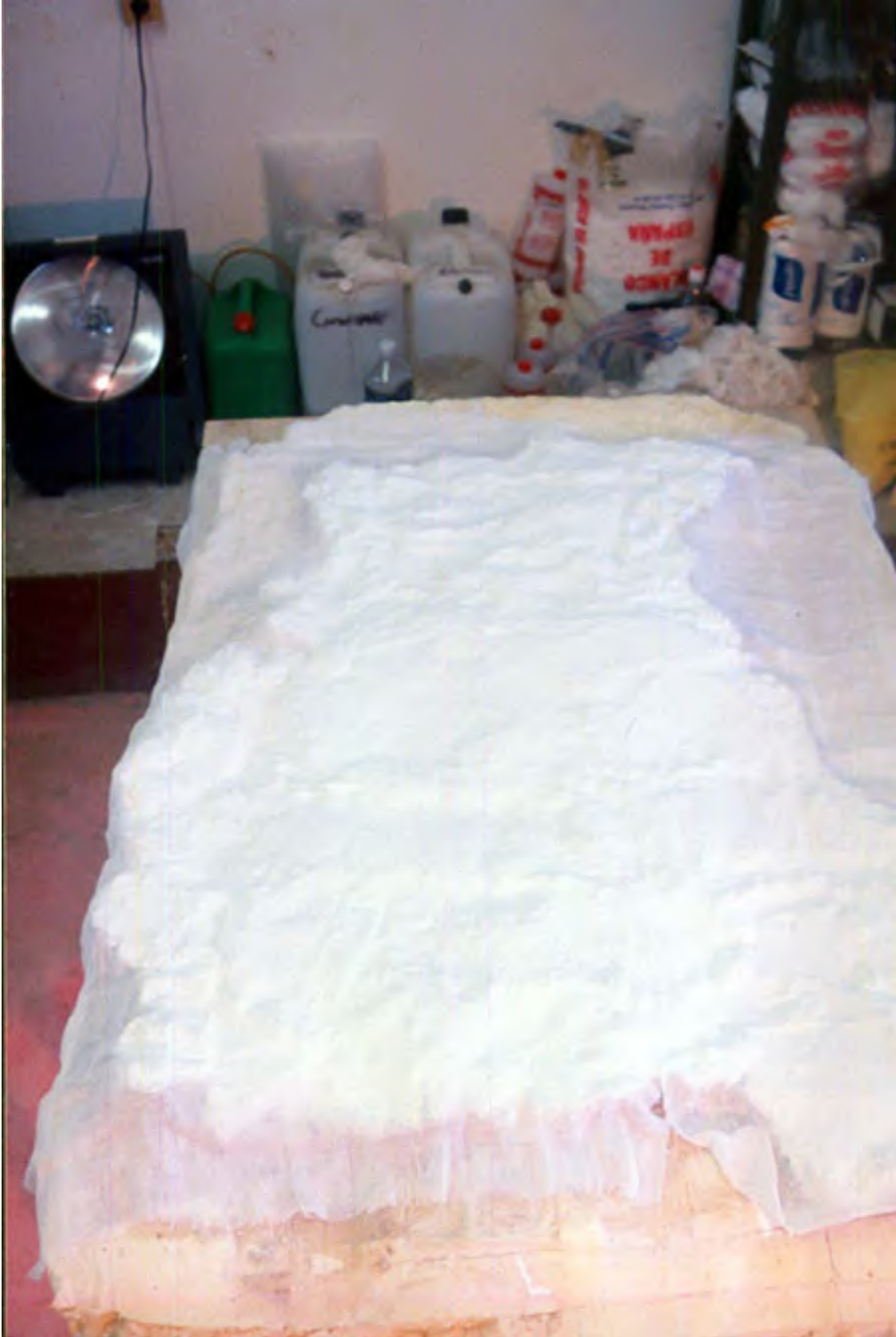
Photo 26. Cheesecloth and calcium caseinate insulating layer
