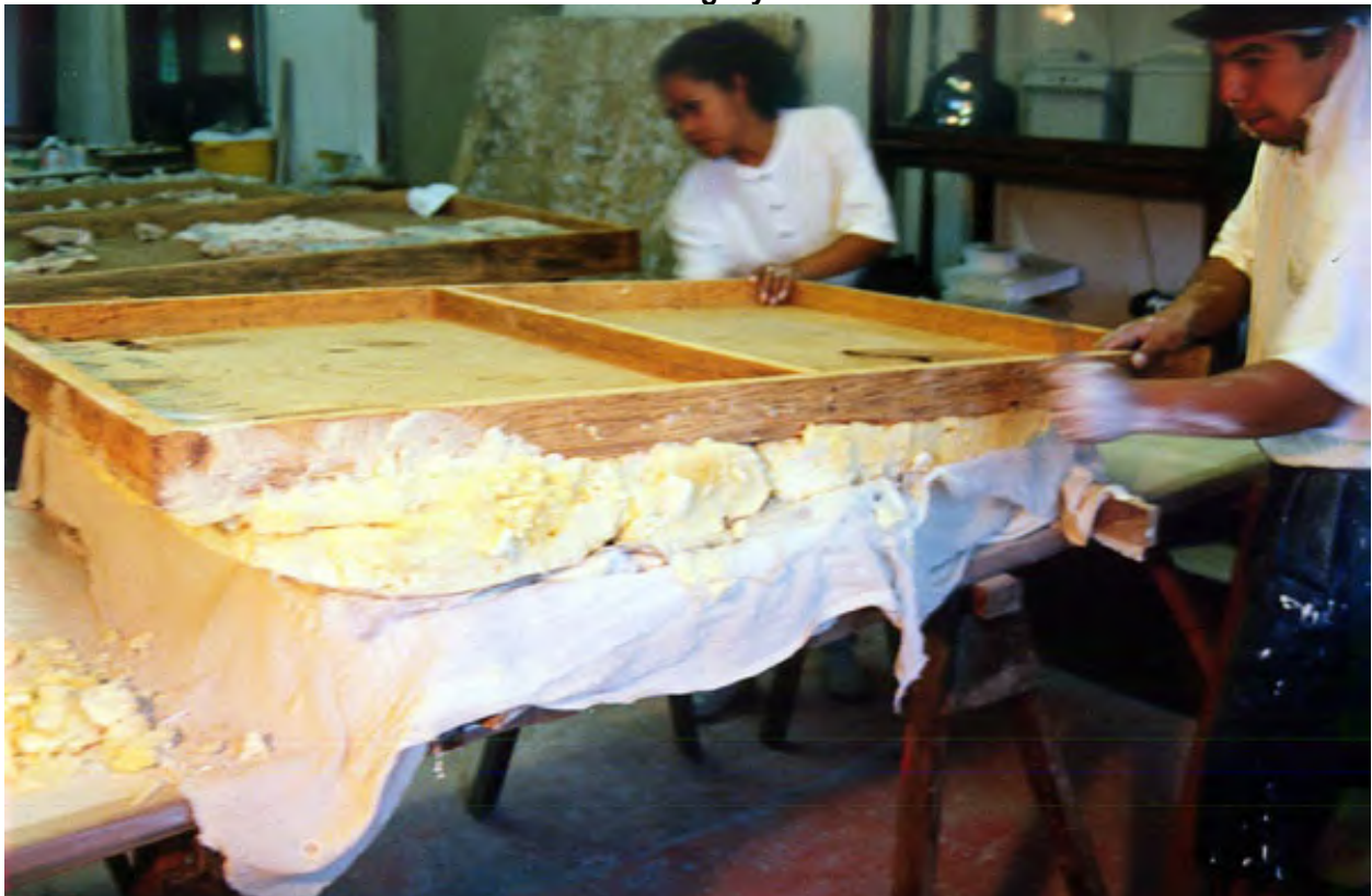
Photo 38. Removal of supporting plank of area detached from wall
