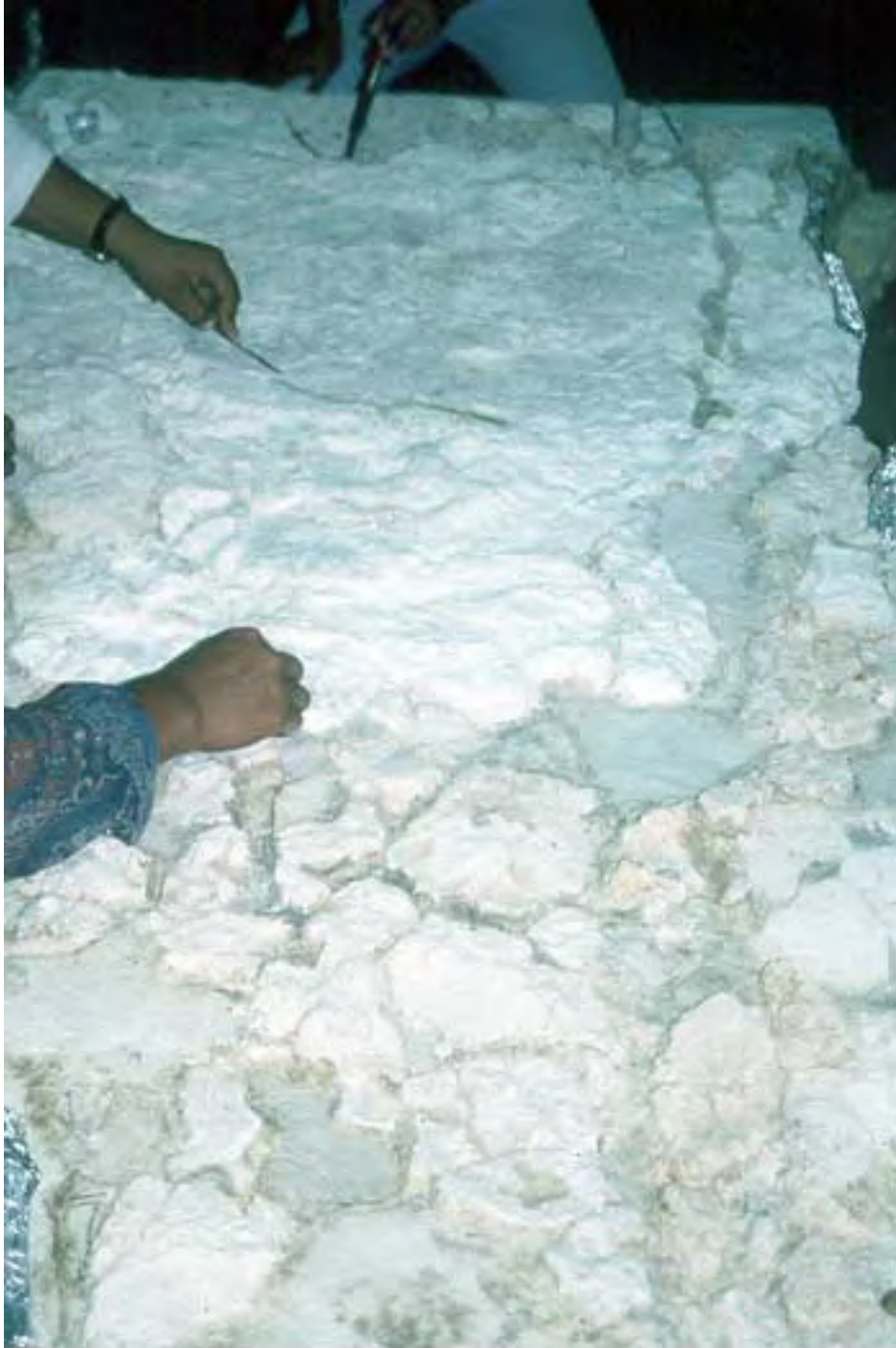
Photo 69. Repairs on the reverse of the stucco panel
