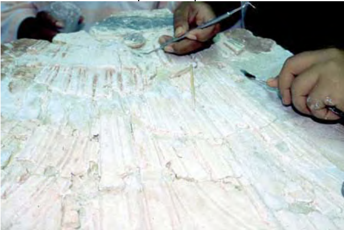
Photo 59. Repairs in joints with ceramic paste
