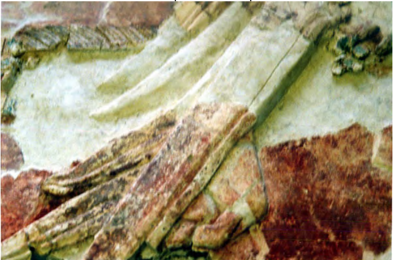
Photo 61. Repairs with ceramic paste
