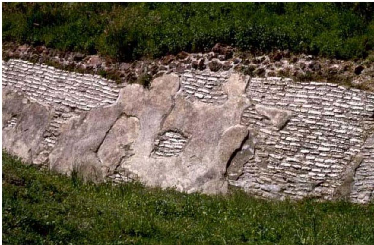
**Photo 26. Cholula, restoration with the use of small stones in the joints to show the reintegrated portions, July 16, 2000.**
