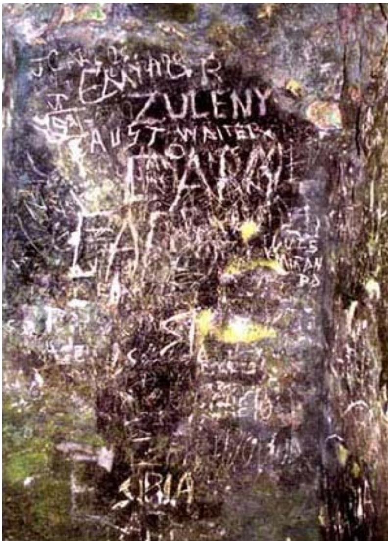
**Photo 56. Tikal, Structure 5D-33-2nd, interior of chamber with modern graffiti on the original stucco. Deterioration here was caused by man and not by humidity.**
