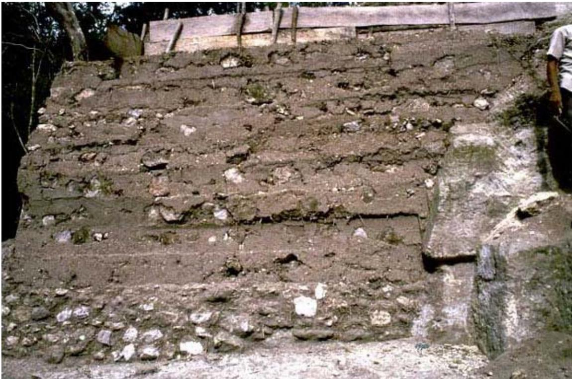
**Photo 25. Yaxhá, detail of experimental restitution of volumes with mud and stones, May 27, 2000.**
