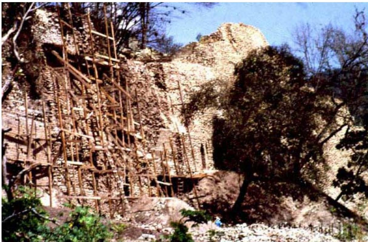
**Photo 64. Copán, archaeological cut, in the process of stabilization. Wooden scaffolds were used throughout the entire work, 1992.**
