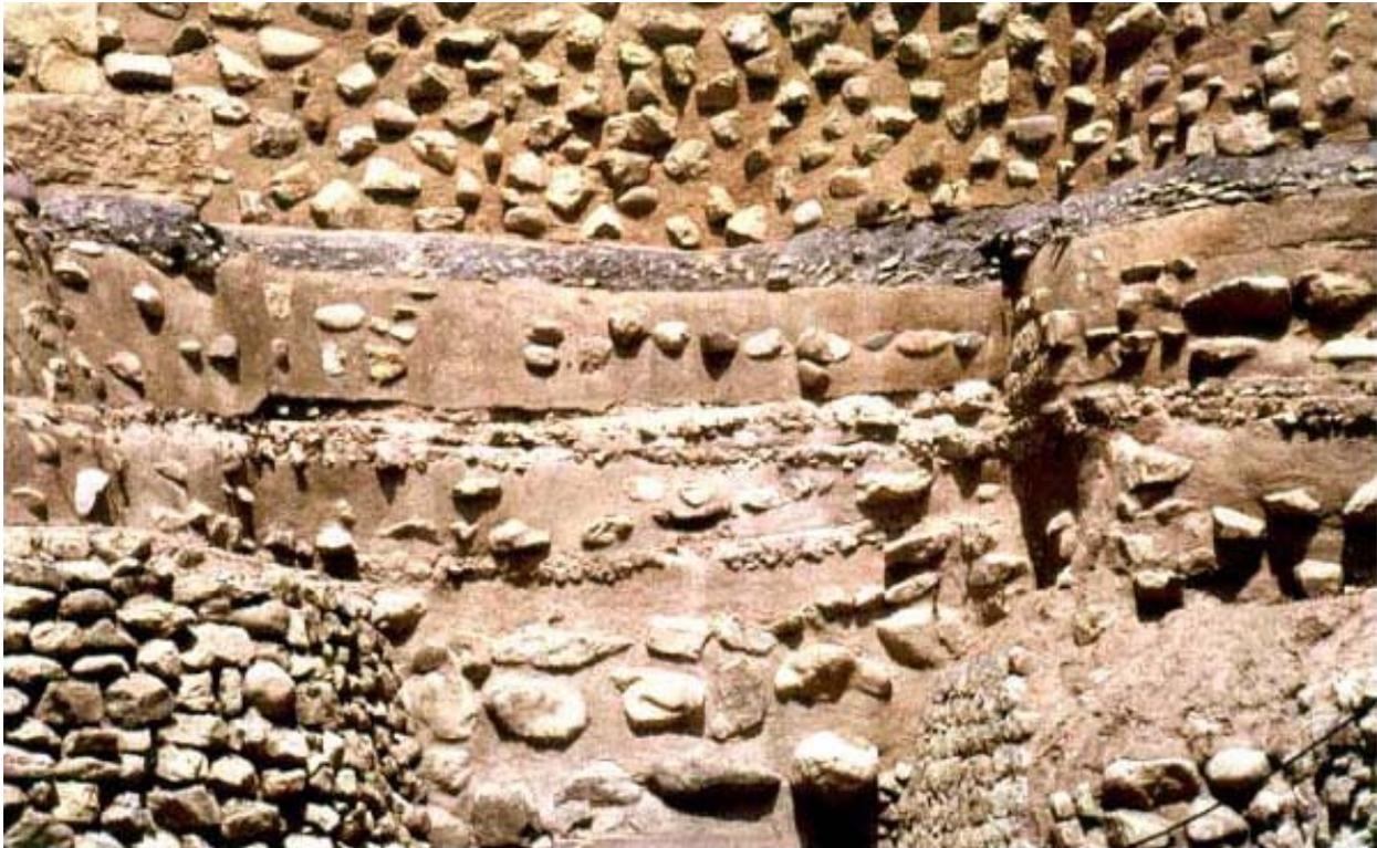
**Photo 60. Copán, showing in detail how the cut was stabilized and cultural strata restored, 1991.**
