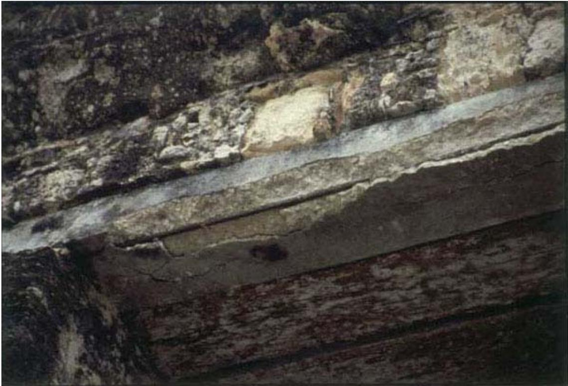
**Photo 14. Tikal, Temple IV. Lintel with deteriorated concrete. May 22, 1991.**
