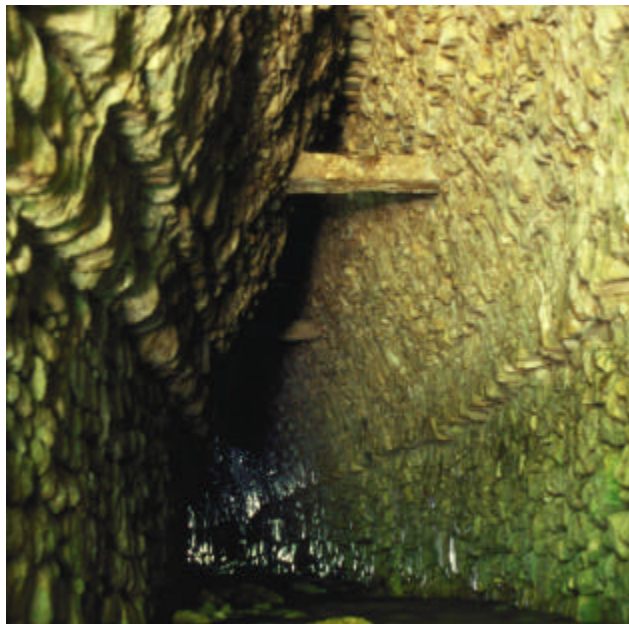
Figure F 2 – An interior view of Palenque's most beautiful aqueduct, OT-A1. Notice the stone support beams found in the corbelled arch.
