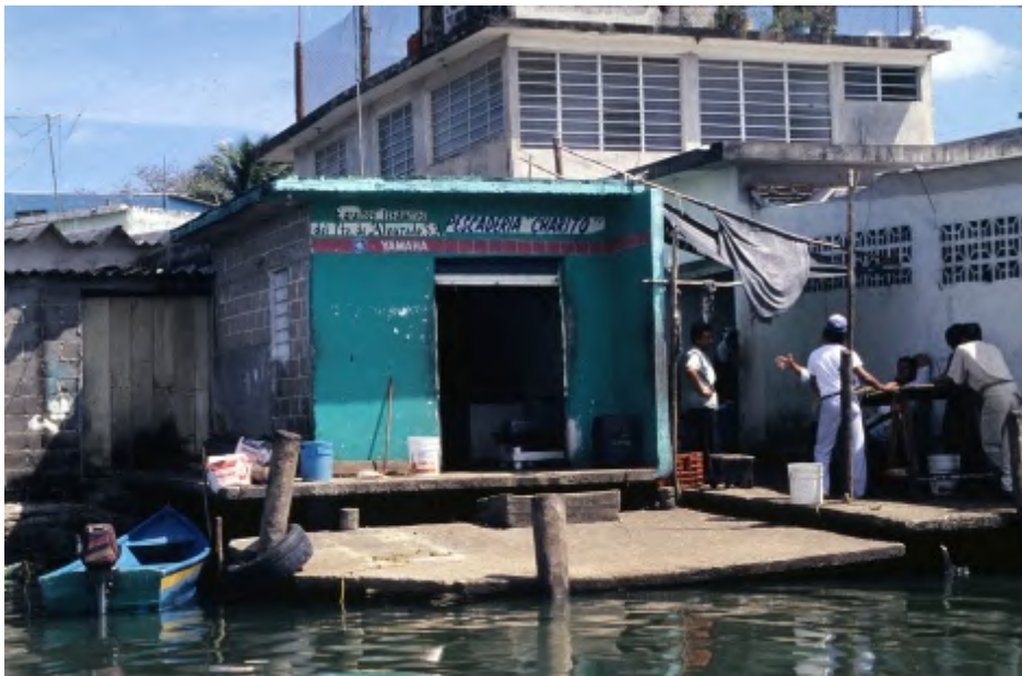
Figure 4.13. One of numerous receiving stations for catches of fresh water fish. Most fish seem to be destined for local consumption and Alvaradeños are fanatics about consuming only fish that are as fresh as possible. "Look that fish in the eye!" takes on a whole new meaning here!
