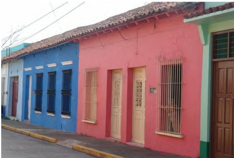
Figure 4.9. A walk around the downtown residential zone is like looking through a kaleidoscope of single story masonry building facades. These simple walls conceal front rooms and corridors leading to interior courtyards and the more private parts of the home. Many families who do not go to the plaza in the evening continue to follow the tradition of moving chairs, especially rocking chairs, out on the sidewalk to enjoy the fresh breeze and socialize with neighbors and passers-by.
