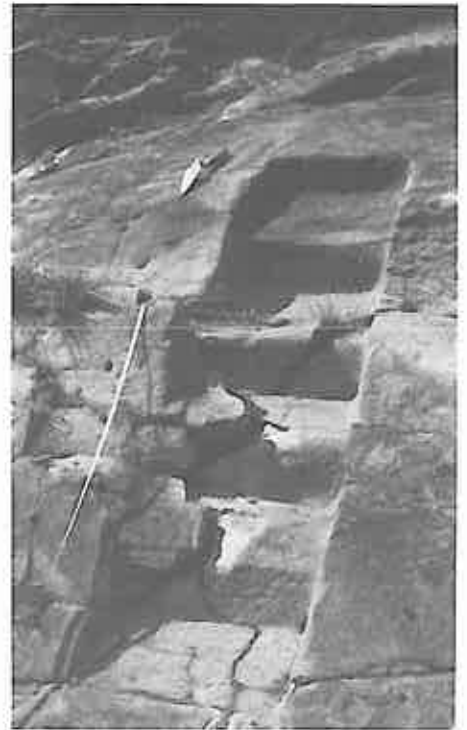
Figure 11.9. MCR-11, lower stairway.
