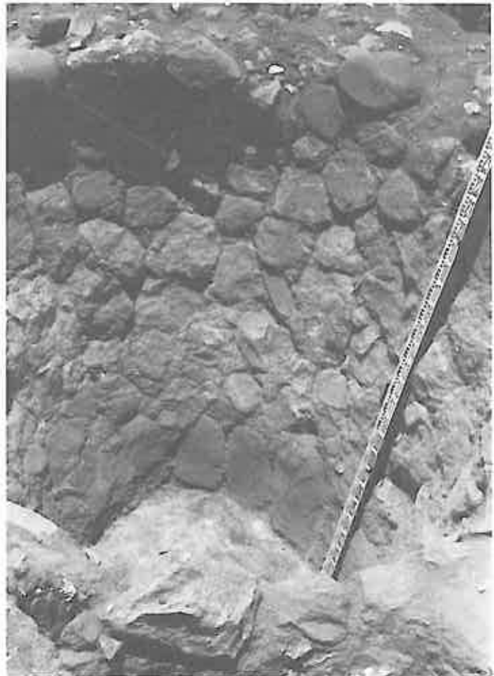
Figure 24.11. Classic lime kiln (T-4 Structure 4) after excavation.
