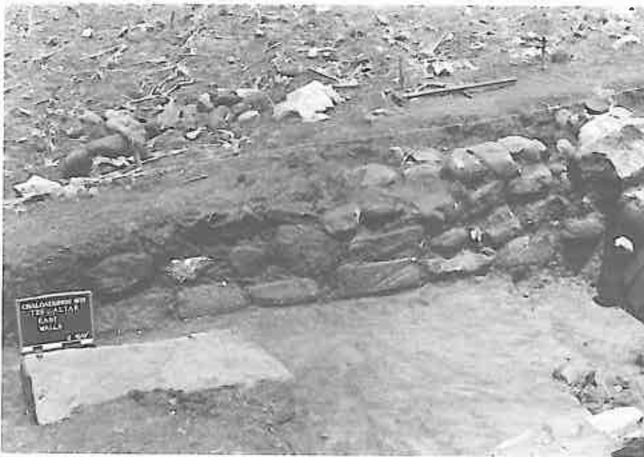
Figure 7.8. Eastern patio wall, construction Stage d.
