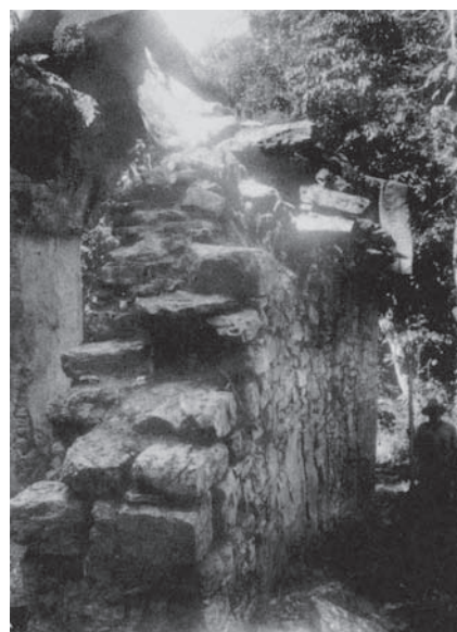
Figure 9.67 Broken section through right end of wall of enclosing building, Structure P-7-1st; squared blocks at lower left and in jamb of doorway.
